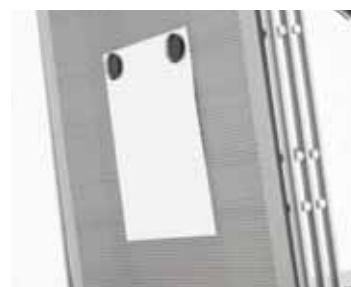
Detail of microperforated steel external closing
